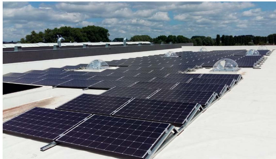
Roof insulation, lightcatchers and solar panels
