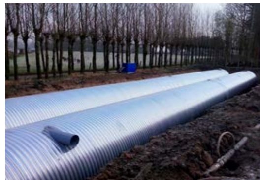
Installation of a rainwater tank
