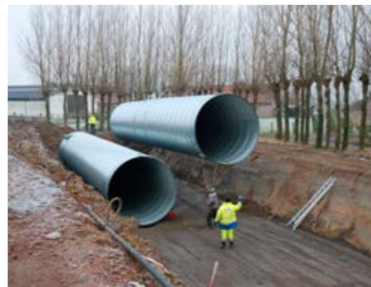
Installation of a rainwater tank
